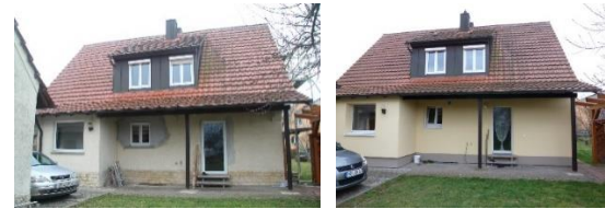
Photos: before renovation after renovation
